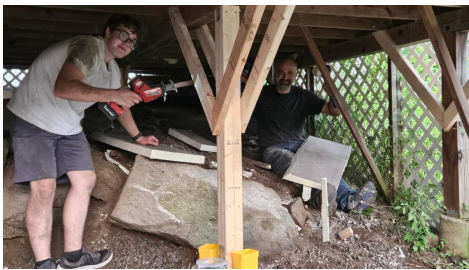
James and Nate reinforce the floor system under the future sacristy!
